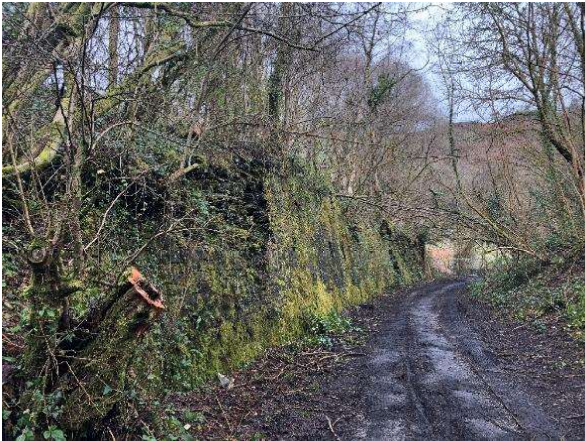
Plate 5: Masonry retaining wall alongside the footpath to the north.
