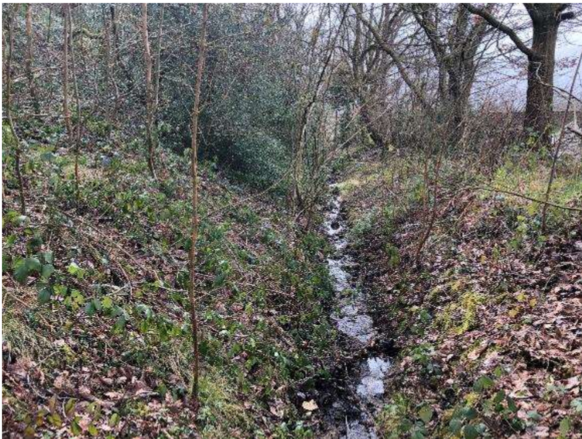
Plate 18: Unlined cut-off ditch running along the toe of the western flank.
