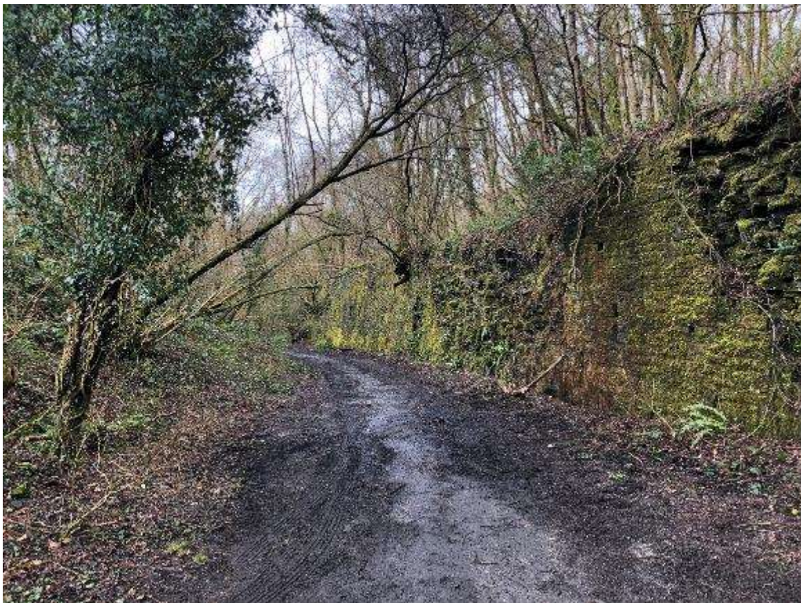
Plate 6: Masonry retaining wall alongside the footpath to the north.
