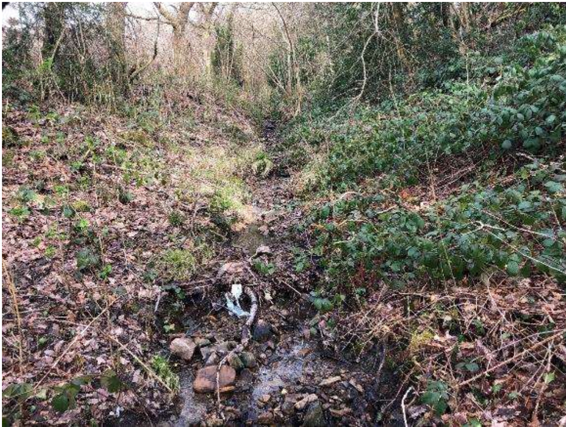
Plate 17: Unlined cut-off ditch running along the toe of the western flank.
