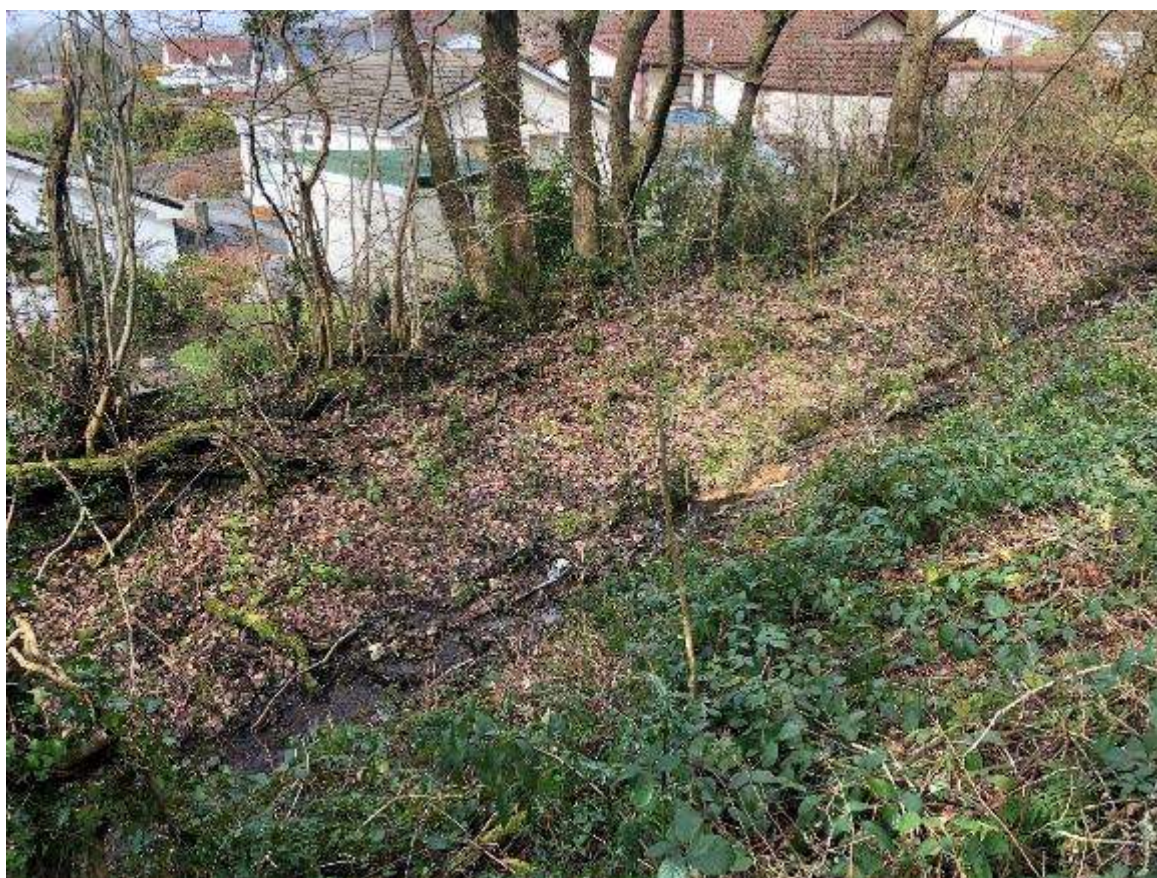
Plate 16: Unlined cut-off ditch running along the toe of the western flank.
